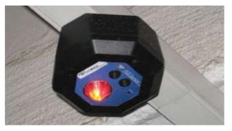
HexBox combo PGS sensor Trunking embedded combo PGS sensor
